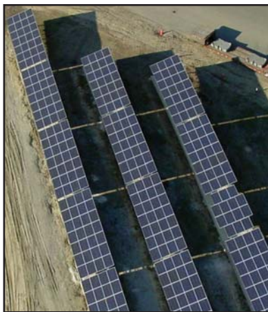
■ A U-LA ground array catches the sun on December 21, when the sun is lowest in the northern hemisphere. The sub-arrays are spaced just far enough to avoid shading.
