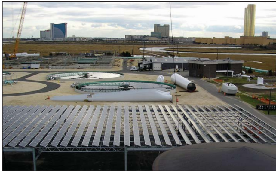
■ Fifty-two rows of PV, each consisting of 18 modules, form a canopy over the carport at the ACUA wastewater treatment plant.
