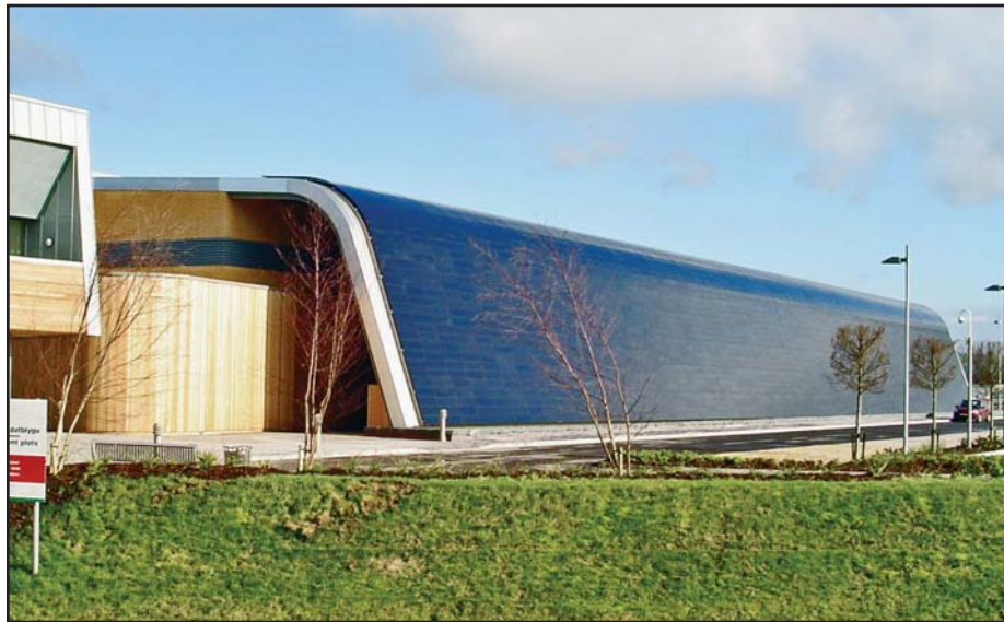
■ The Solar Wall forms a sweeping façade covering the entire south face of the Welsh Development Agency “Technium” in St. Asaph.
