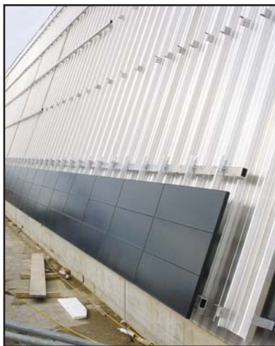
■ Hidden SolarMount® bottom-mounting clips secure modules from the rear, giving the array the smooth exterior face sought by its designers.
