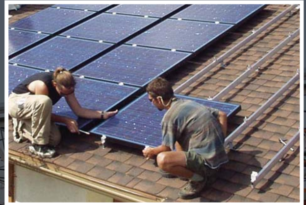
■ Top mounting: Attach modules one-by-one to installed rails.
