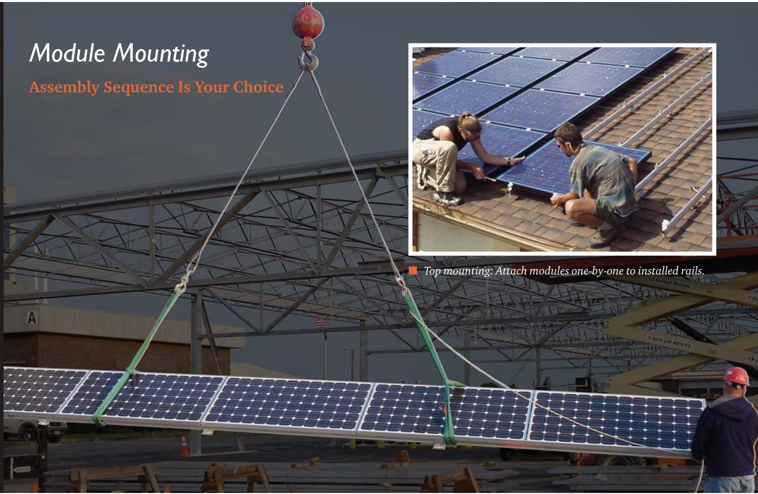
■ Bottom mounting: Preassemble full rows before final installation (standard and HD rail only).
